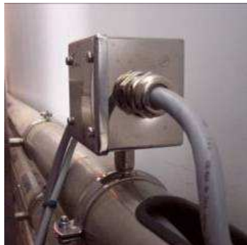
Typical IP65 Junction Box
