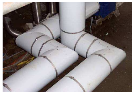
Figure 2 - Typical Inditherm Heating under Fixed Cladding
